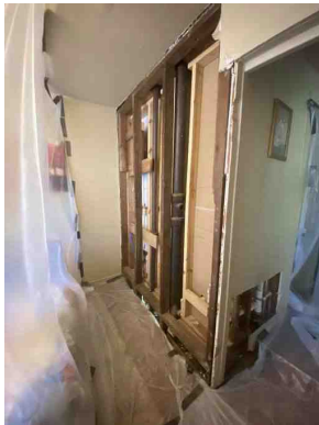
Unit D Water Damage Repair
