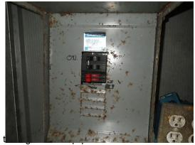
circuit breakers do not trip about 25% of the time when exposed to overcurrent - risking overheating, fire and other hazards. The failure rate of competitive-brand circuit breakers is much less than 1%. Further evaluation of this panel by a qualified electrician is recommended.
