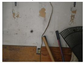
Wires entering switch panels are not protected by bushings or wire clamps as required, making them subject to abrasion damage on knockout edges.
