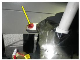
The dryer filter on refrigerant tubing of the south HVAC system is heavily rusted. Repair is recommended prior to rust-through that can cause loss of refrigerant.
