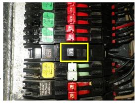
The double-pole 40-ampere breaker at the bottom of the panel has a poor connection with the bus bar, creating risk of resistance heating.
