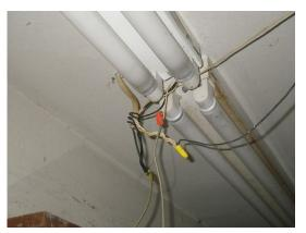
Non-metallic sheathed wires surface-mounted on the south and east interior wall of the garage are not rated for unprotected installation and are subject to damage from stored items. The wires should be contained in conduit or routed within the wall cavity.
