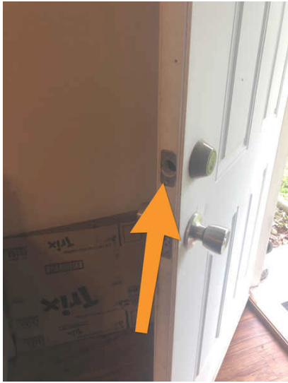
Front Exterior Wall
