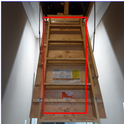
D. Item 1(Picture) Pull down stairs
