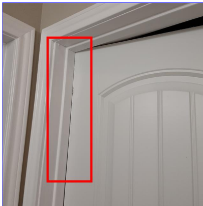
G. Item 4(Picture) Master closet
