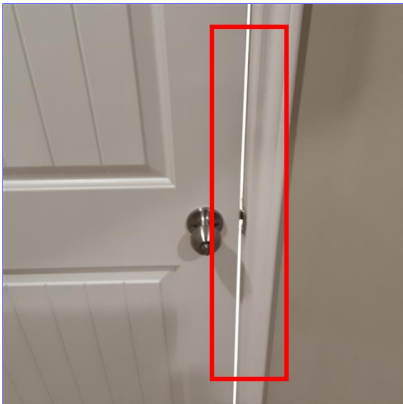
G. Item 2(Picture) Door to garage
