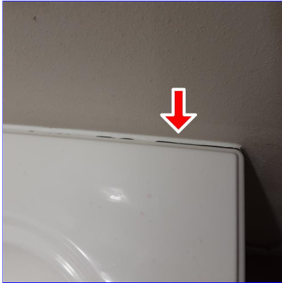
E. Item 2(Picture) Master bathroom
