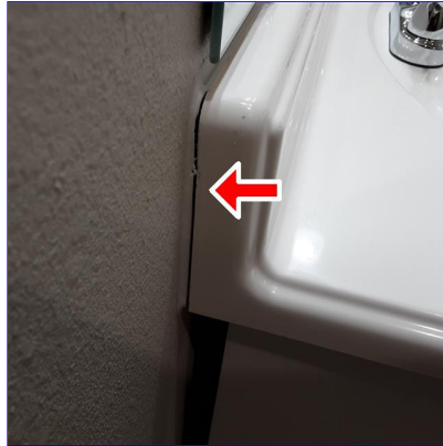
E. Item 3(Picture) Master bathroom
