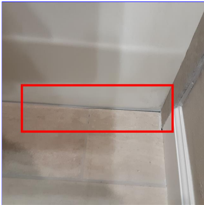
F. Item 1(Picture) Master bathroom at tub
