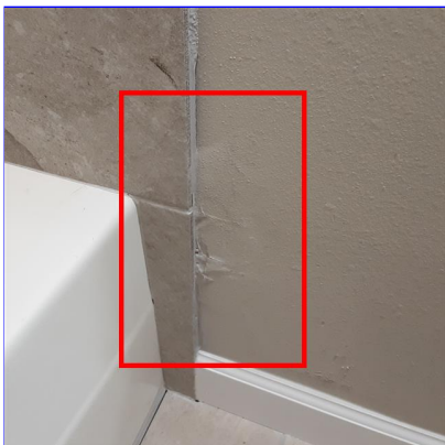
E. Item 1(Picture) Master bathroom
