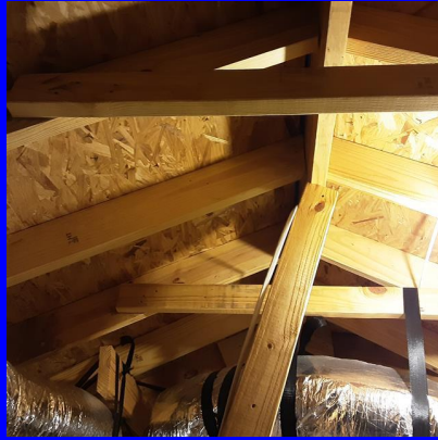
Stick built 2x6 rafters
