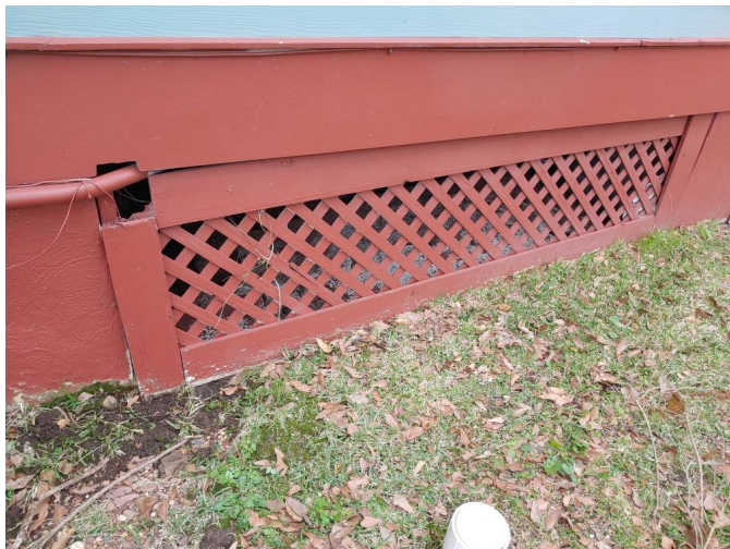
G. Wood to Ground contact on vents
