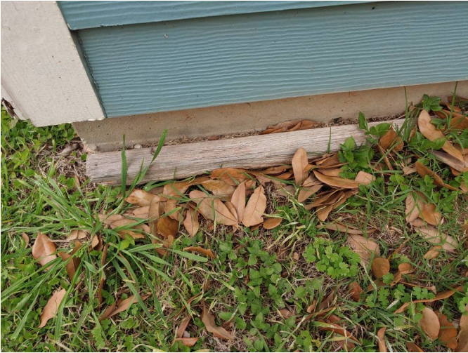
I. Form boards left in place
