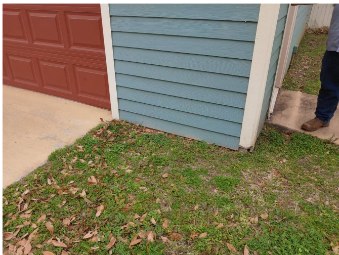
L. Ground High on slab
