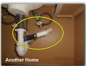
124The main drain line is PVC which is good.
