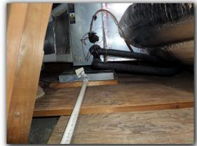
135The ducts must be elevated and supported from the rafters.
