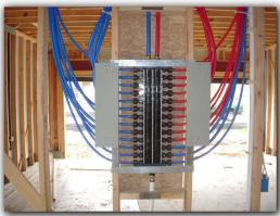
157PEX (or *cross linked polyethylene*) is part of a water supply piping system that has several advantages over metal pipe (copper, iron, lead) or rigid plastic pipe (PVC, CPVC, ABS) systems. It is flexible, resistant to scale and chlorine, doesn't corrode or develop pinholes, is faster to install than metal or rigid plastic, and has fewer connections and fittings.
