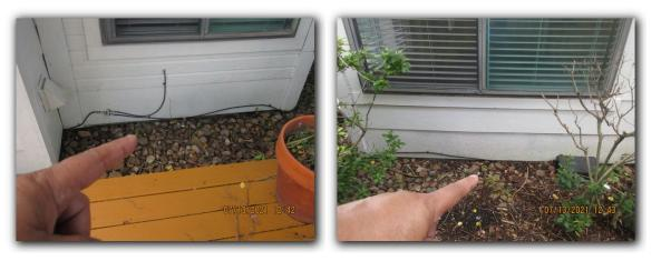
9. Note: Any area where the ground or grade does not slope away from the structure is to be considered an area of improper drainage. Six inches per 10 feet.
