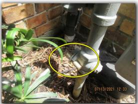
140Gas meter was not bonded as required by code
