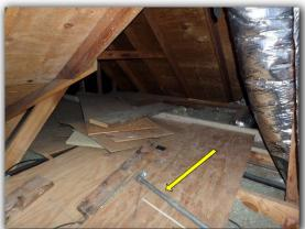
152.If the home has galvanize water lines they should be replaced in the near future before they fail as they are failing all over the U.S. due to age.
