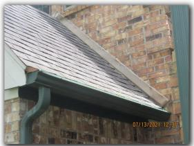
39. Missing metal flashing above arched window trim as per IRC code R-703.8.1.4 & R-703.1
