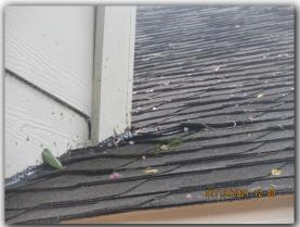
19. The plumbing roof jacks are lead and are in good condition but the base needs to be sealed and secured.
