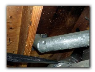
171The vent pipe is a Type B with cap and collar as per code.
