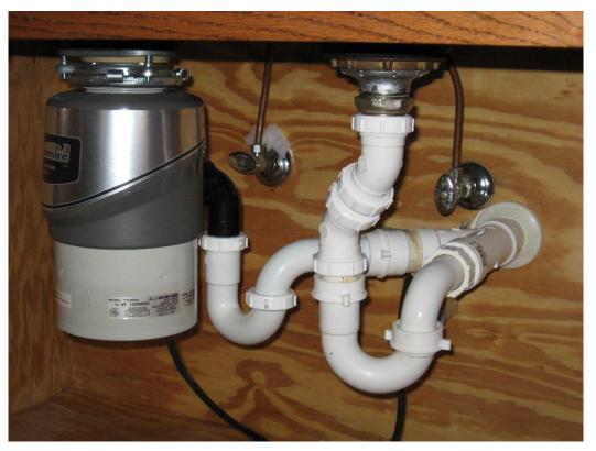
205When the proper installation is completed, the drains will then work as intended since there is a full pipe diameter drain from each sink.
