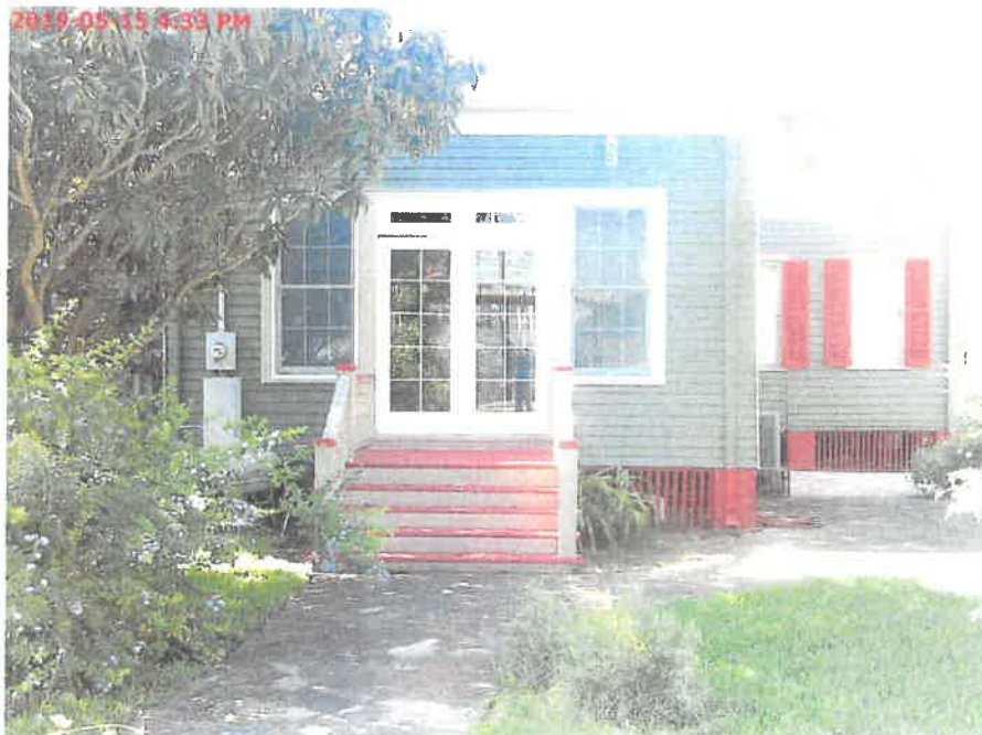
Picture Taken: May 15, 2019 REAR VIEW
