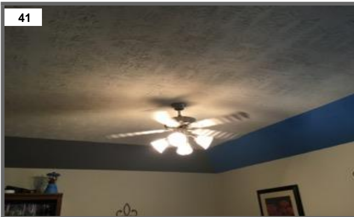
left upstairs bedroom
