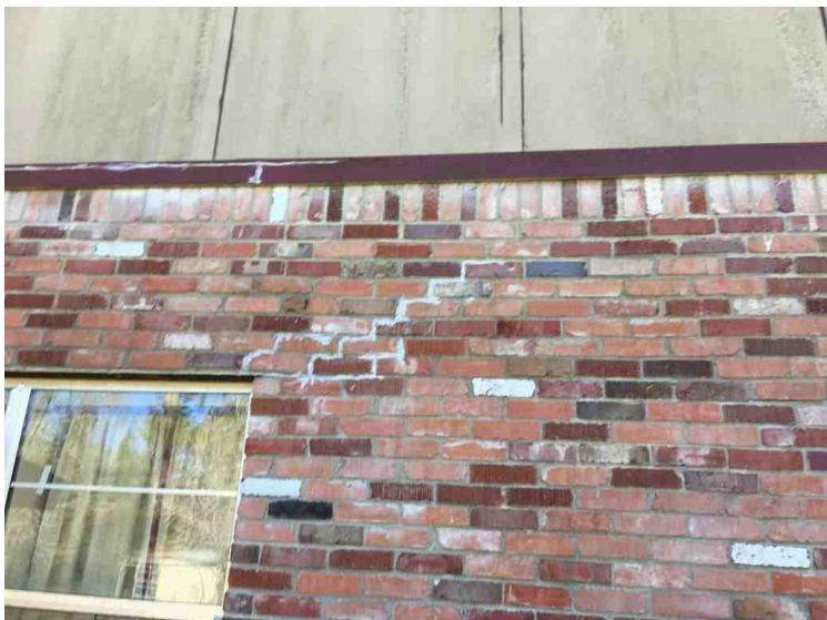
Settlement Crack
