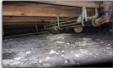
Crawl Space viewed From: Crawled Structure
