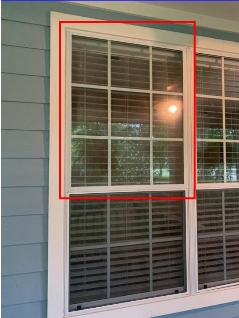
H. Photo 1(Picture) One of the front porch area window seals appears to be compromised, as suggested by condensate and mineral deposits built up between the double panes of glass.
