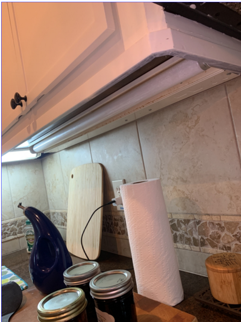
B. Photo 1(Picture) One of the kitchen under-cabinet lights did not turn on with the switch.
