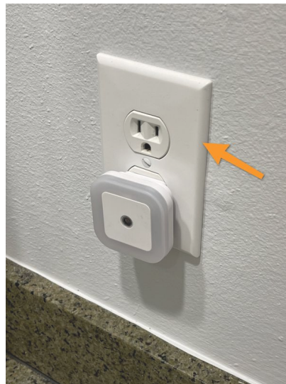
1st Floor Bathroom
