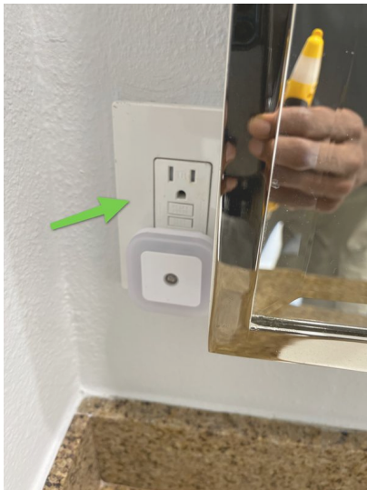
Master bathroom GFCI reset switch is interconnected to all bathroom GFCI outlets
