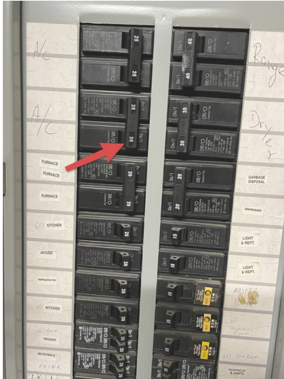
Max breaker 30amp, 35amp installed
