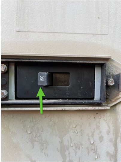
Electrical service to home is 150amps
