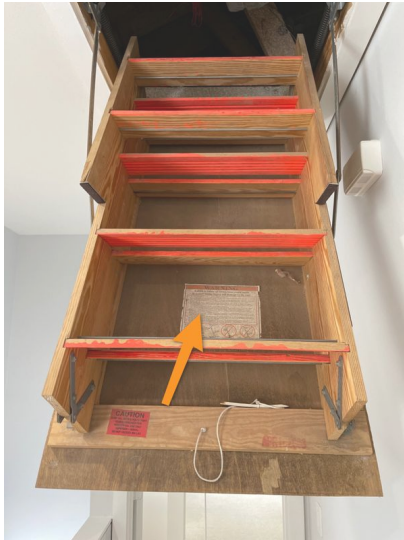
3rd Floor- attic
