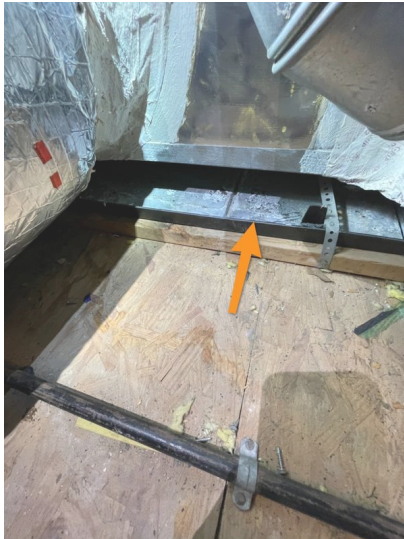
Attic- right side unit
