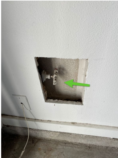
Inside garage right wall
