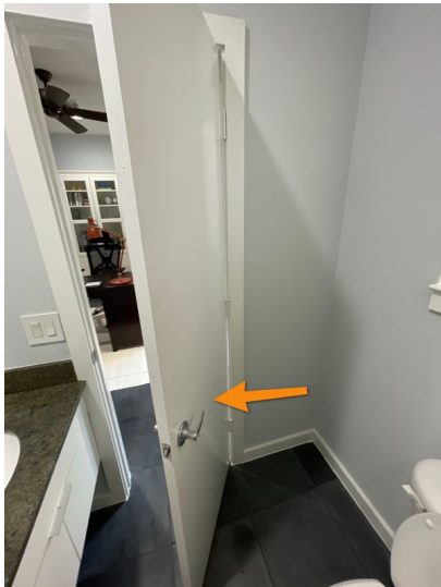
1st Floor Bathroom
