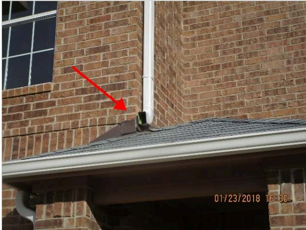
Downspout terminating onto a lower roof
