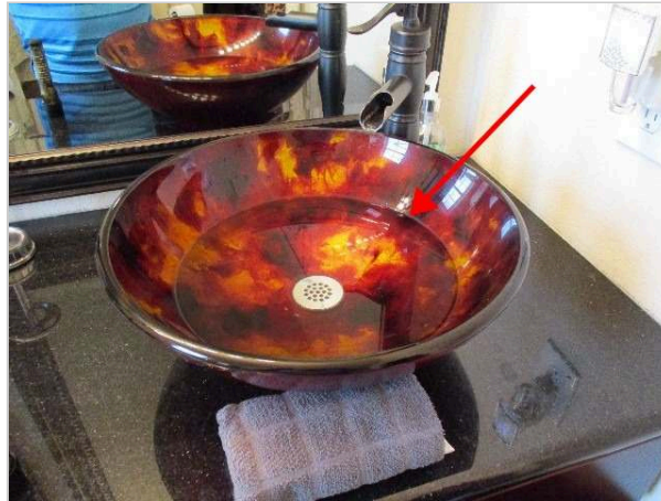
Sink slow to drain
