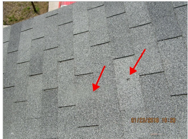
Damage / Bruised shingles
