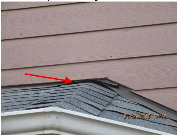
Raised flashing
