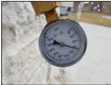
Water pressure at front elevation
