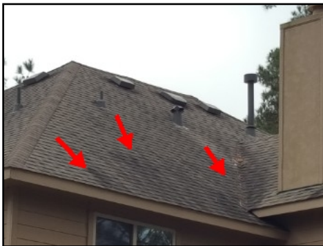
Airborne algae present on shingles
