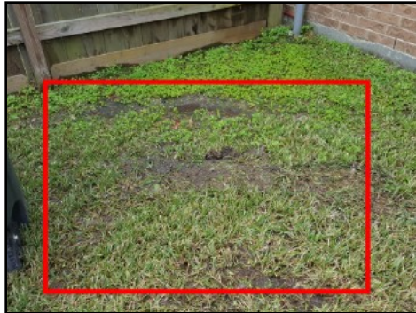
Excessive moisture at rear right elevation
