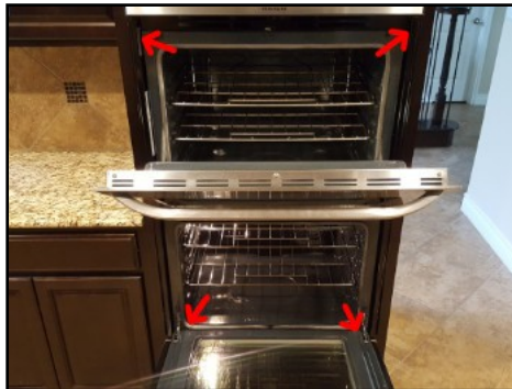
Double oven not secure in place
