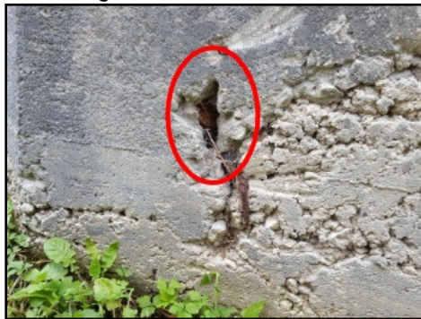
Exposed fixed end of tension cable
