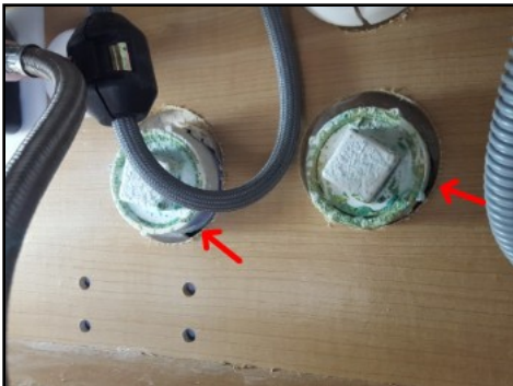
Seal all interior penetrations
