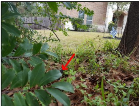
Water meter location
