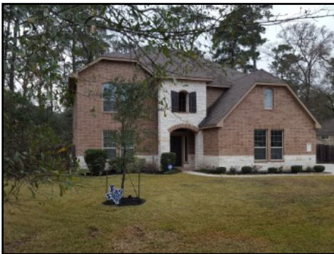
Left elevation of home
