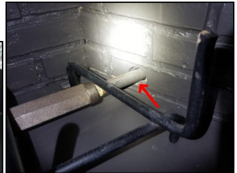
Seal gas line through fireplace wall
