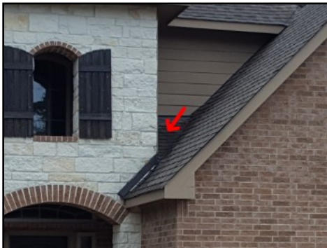
Monitor "trap" area in roof design
