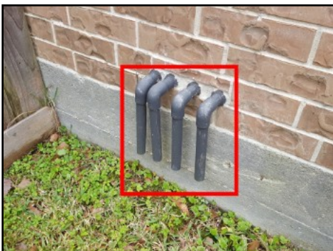
Drain line termination at left elevation
