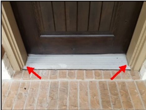
Keep door thresholds/jambs sealed
