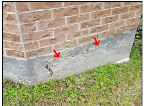
Exposed aggregate at rear elevation
