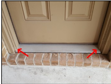
Seal door thresholds/jambs
