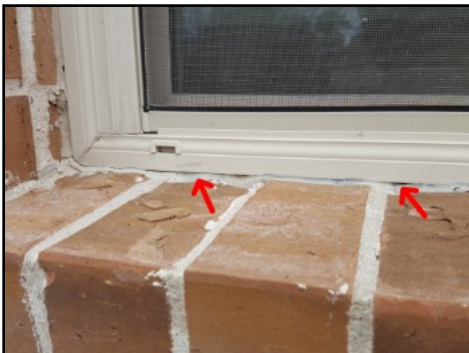
Seal exterior window frame at front elevation
