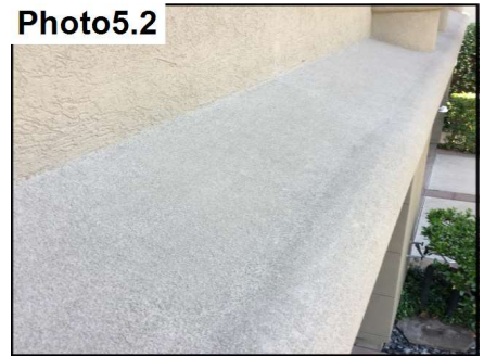
Apply four coats of elastomeric at semi-flat wall.
