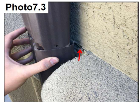
Photo7.3 Seal / Repair cracks as needed.
