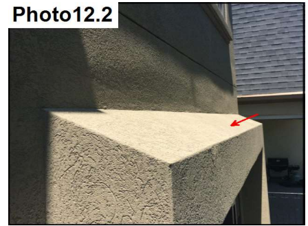
Install a metal cap at pitched wall.
