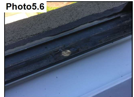
Alarm sensors are present at windows.
