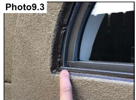
Windows are adequately sealed.
