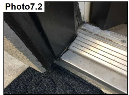
Photo7.2 Reseal door miters as needed.
