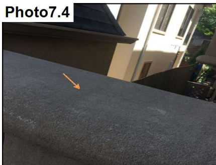
Photo7.4 Install a metal cap at flat wall.
