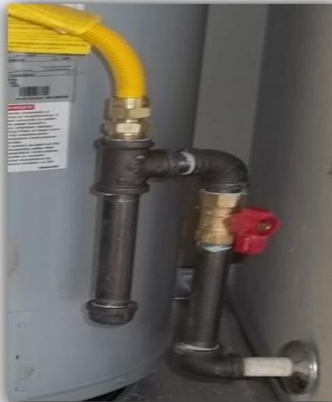
Samples of correct sediment trap installations
