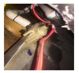
The overflow pan under the evaporator coil had rust in the pan, apparently from water overflowing the condensate drain line into the overflow pan. No water was in the pan at the time of the inspection, but, since we only ran the unit for a few minutes, it is recommended that the drain line be checked by an air conditioning service company. **Obtain Cost Estimate**
