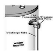
The relief valve was not operationally checked at the time of the inspection. Valves typically do not reseat properly when they are operated, which causes the valves to leak. It is best to replace the relief valve every 2-3 years. (Information)
