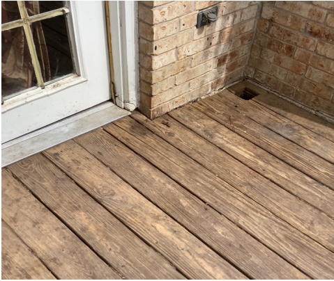
Vertically drill exterior attached slabs and treat
