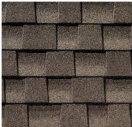
Roof. Weathered Wood Per Community Guidelines
