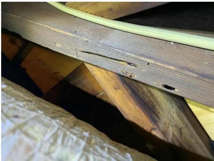
Evidence of wood boring beetles
