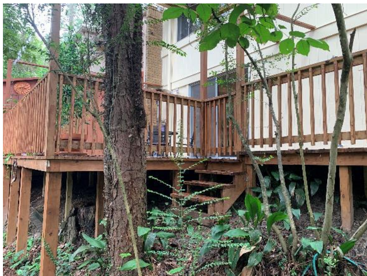
Wood deck in contact with the ground and the structure
