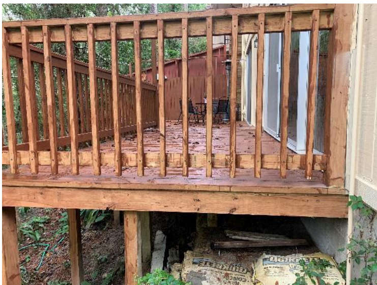
Wood deck in contact with the ground and the structure
