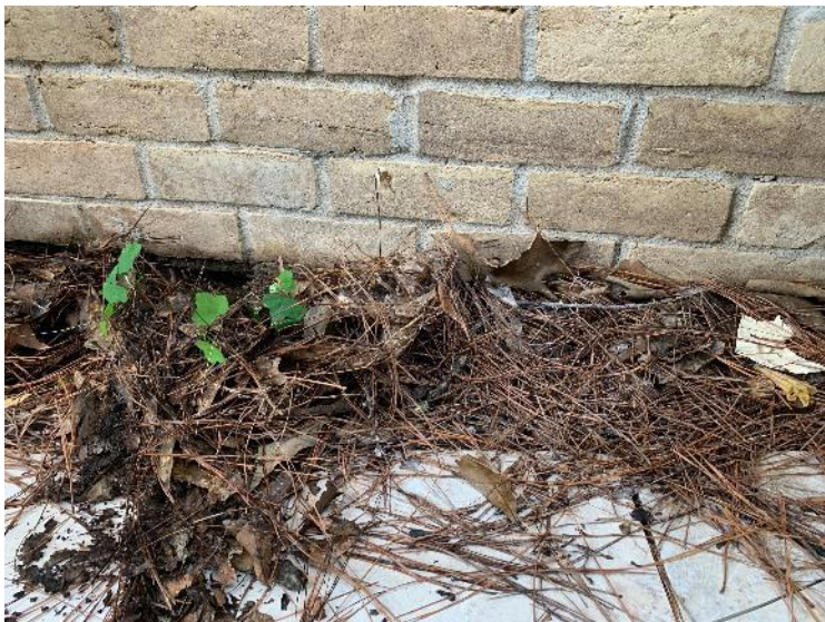
Debris observed near the structure and should be removed
