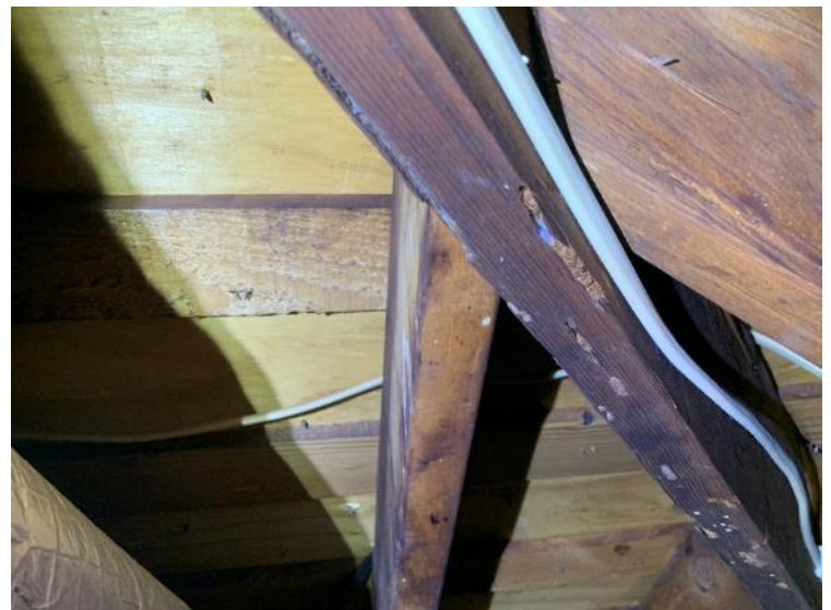
Evidence of wood boring beetles
