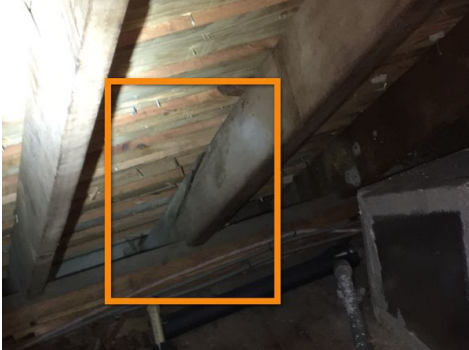
West side of the attic
