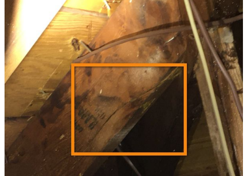
South area of the attic
