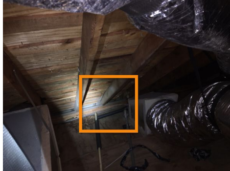
West side of the attic
