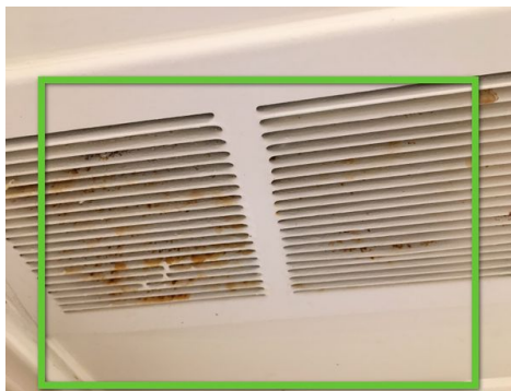
Small room near the kitchen
