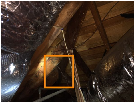
South area of the attic
