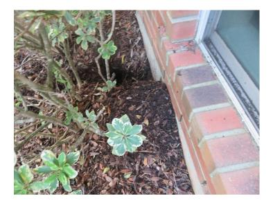
Along the rear wall of the house, the gap between the pool deck and house should be properly encapsulated.
