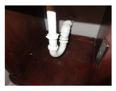
> The right sink in the Primary bathroom does not readily drain.
