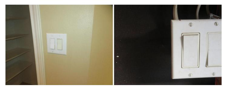
> All light switches and outlets are required to be provided safety cover plates.
