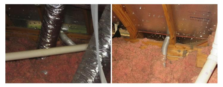
> Exhaust fan ductwork in the attic rising through the roof deck should be sealed.
