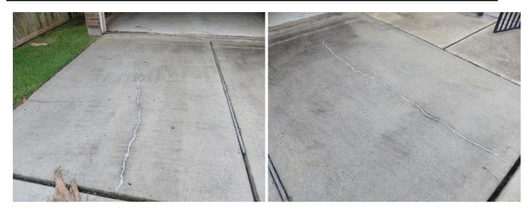
> The driveway has lost its expansion joint material.
