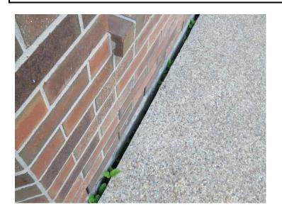
At the rear of the garage soils are installed too high against the rear framing and wall surfaces. Dirt and moisture is penetrating into the garage.
