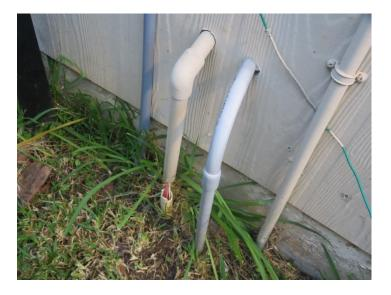
Sprinkler heads in Zone 3 (right rear home corner) and at the rear flower bed behind the pool lacked water spray and displayed leakage.
