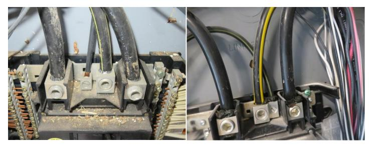
The Main service entrance exhibits Neutral wires that have been double lugged (connected together) at the Neutral bar. This installation can cause an overheating condition between the two or more wires. Each Neutral wire should be separated and assigned its own lug for connection.
