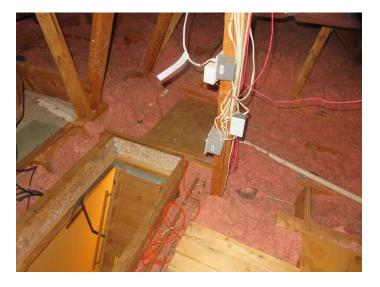
> The main attic floor displays a hole creating a safety hazard.
