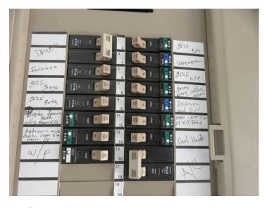
4 As of approximately 1/1/2008, all electrical fixtures, outlets, switches and smoke detectors in the home wired to single-pole 15 or 20 AMP circuit breakers {3902.11/IRC}, other than those apparatus protected by GFCI or GFCI/AFCI combination safety device, are required to be wired to AFCI safety circuit breakers in the main panel.
