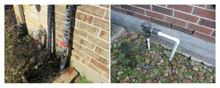
The sprinkler system appears to lack a rain sensor that acts as an automatic shut-off during rainy and wet periods.
