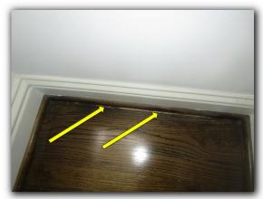
There are cracks beginning to form at the corners of the tray ceiling in the master bedroom.
