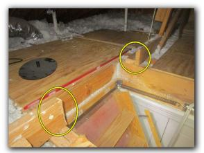
There is a required minimum 24" wide, unobstructed walkway to all attic equipment. The walkway is obstructed / inadequate, creating a potential trip hazard (in the apartment attic).
