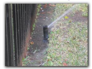
There are sprinkler heads that spray the sidewalk and home at more than one location. The sprinkler heads may require adjustment. Spraying directly onto the home can lead to moisture penetration.
