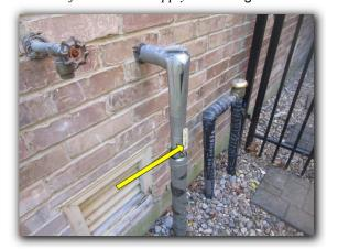
Static water pressure reading: 52 psi Comments: Type: **PVC & PEX**
