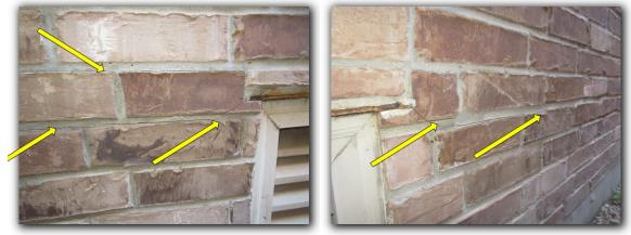
There is a mortar joint crack at the front right corner of the front porch.
