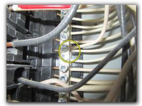
There is no anti oxidant paste on the aluminum service wires at the main lugs in the garage panel.
