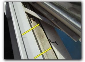
There is evidence of wood rot / deterioration at the front right bedroom window. There are signs of a multitude of ladybugs at this location.
