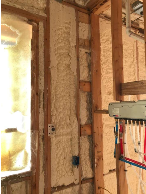
Spray Foam through home and in between floors.
