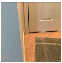
• Under todays standards the garage walk-in door should have spring loaded hinges and be self closing. Its considered a fire door. Consider updating or repairs. (Garage)
