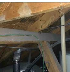
• Dryer vent appears to be installed to vent outside as required. All dryer vents should be kept clear and clean. This is very important if its a vertical vent. Lint build-up can be a fire hazard. Inside the vent pipe was not inspected.
