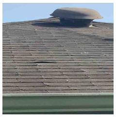
• Ridges or Waves visible in the roofing, It could be poorly installed roof materials, raised / poorly supported sheeting under the shingles or issues with rafters/ truss. Monitor and Maintain as needed.
