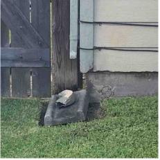
• Effective Grading and Draining should be maintain around the structure. Install gutters and down spouts when needed, use under ground drain systems when needed. Keep Soil/Mulch/Rock 4-inches below brick, 6-inches below siding to help keep water and insect access to the home. These are important to help keep the moisture content of the as stable as possible, helping the foundation support the home.
