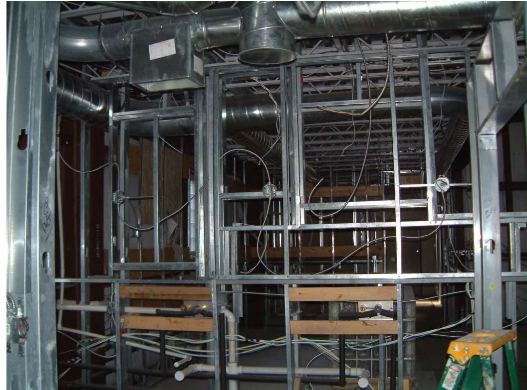
Interior wall construction looking from inside master bathroom toward kitchen area.
