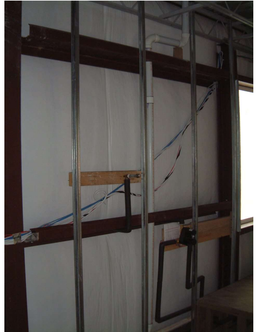
Typical Routing of Piping and Electrical Wiring before Batt Insulation is Installed.
