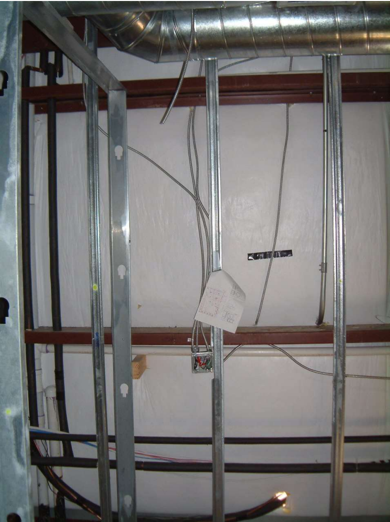
Typical Routing of Piping and Electrical Wiring before Batt Insulation is Installed.
