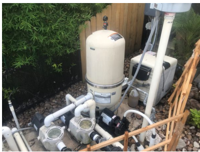
Pump Types:: Circulation, Booster, Waterfall
