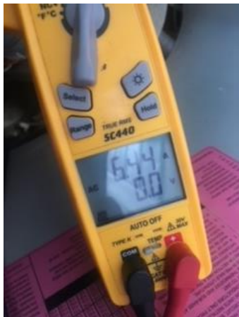
Compressor rated load amp.
