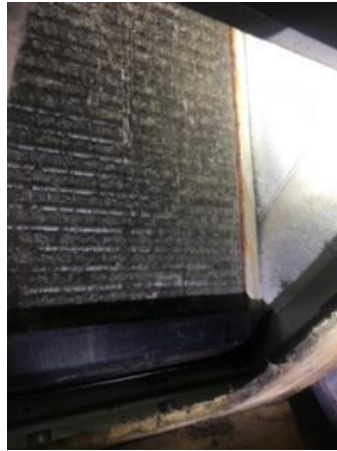
Clean evaporator coil.
