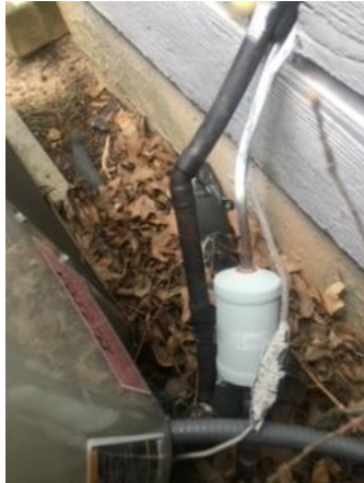
Insulate suction line at condenser.
