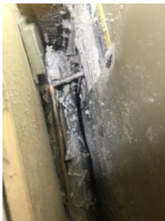
Insulate and tape suction line.
