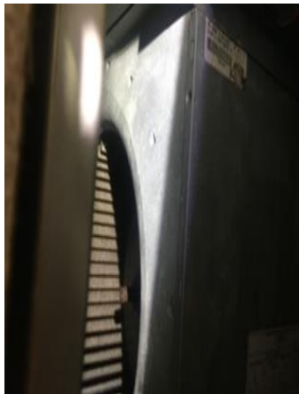
Remove and clean blower wheel.
