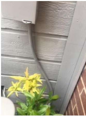
Secure electrical whip.
