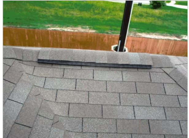
Roof view - rear side
