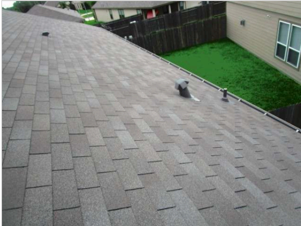
Roof view - Right side
