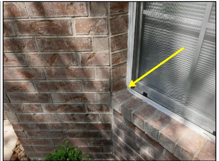
SEAL DETERIORATION
