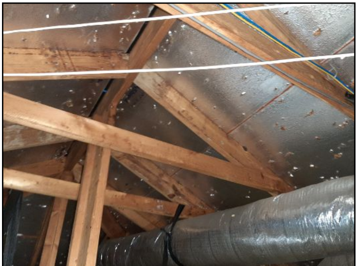
RADIANT BARRIER PRESENT
