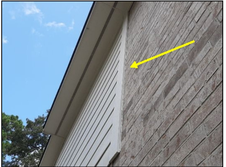
SEAL DETERIORATION
