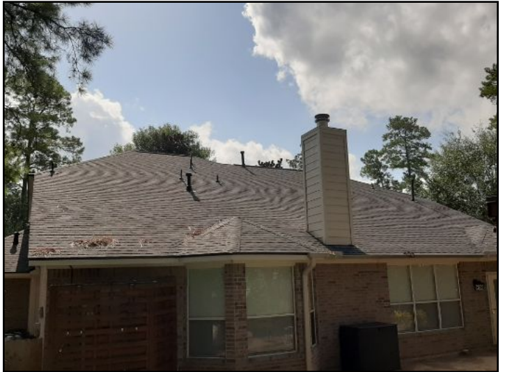
ROOF COVERING; BACK
