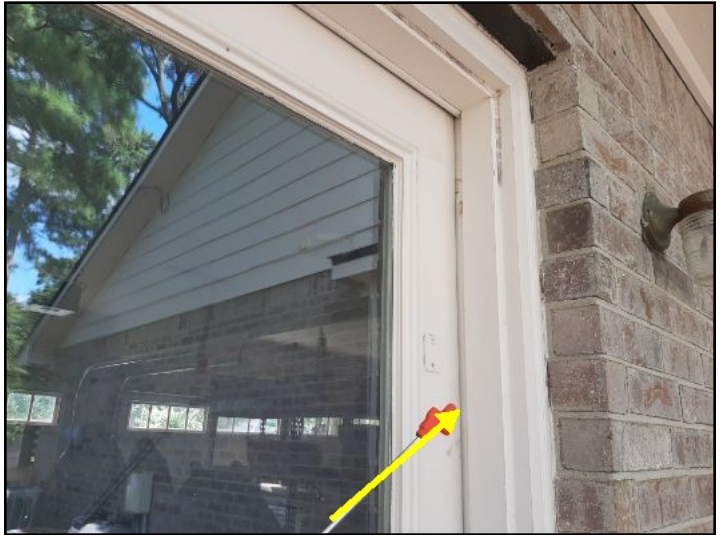
MISSING WEATHERSTRIPPING
