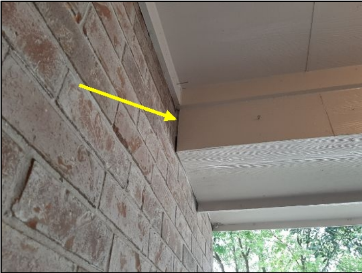
SEAL DETERIORATION
