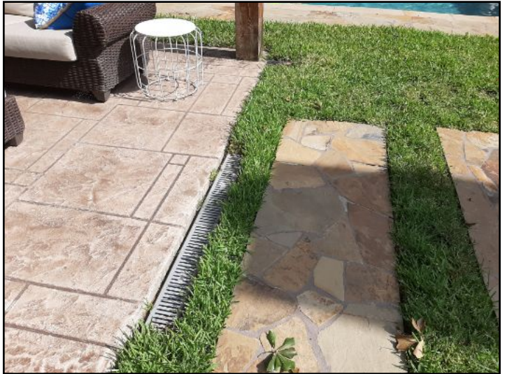
UNDERGROUND DRAINAGE PRESENT OK
