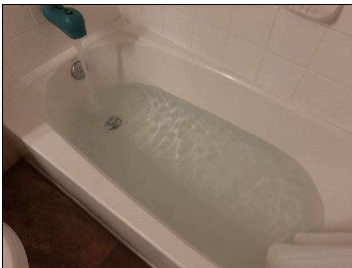
SINK / TUB FILLED AND TESTED
