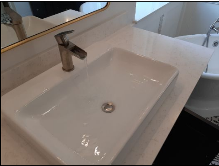
SINK / TUB FILLED AND TESTED
