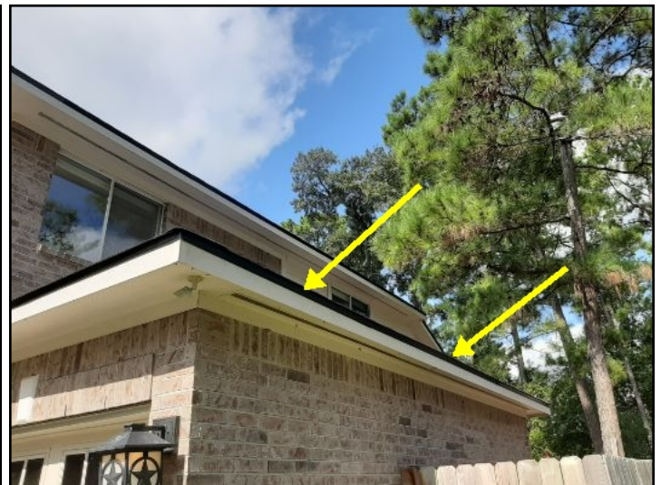
NO GUTTER SECTIONS
