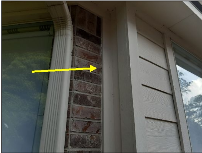
SEAL DETERIORATION
