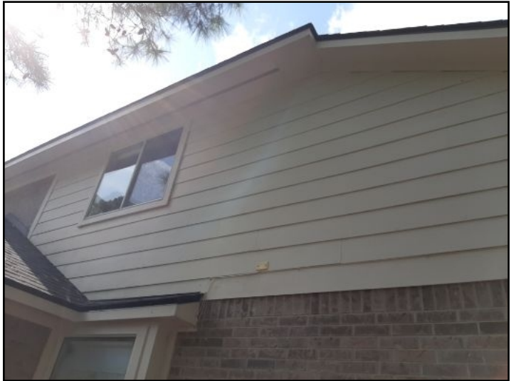
SIDING OVERALL OK
