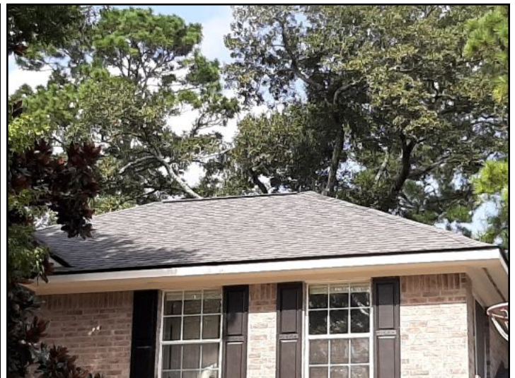
ROOF COVERING; FRONT
