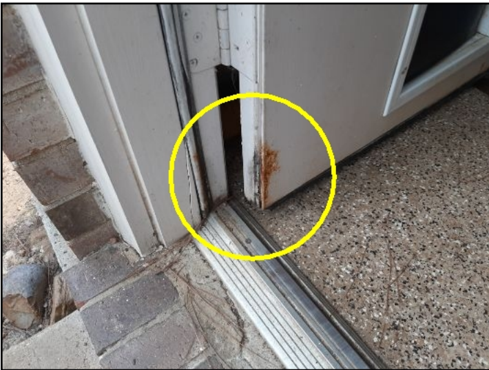
MINIMAL DETERIORATION AT DOOR
