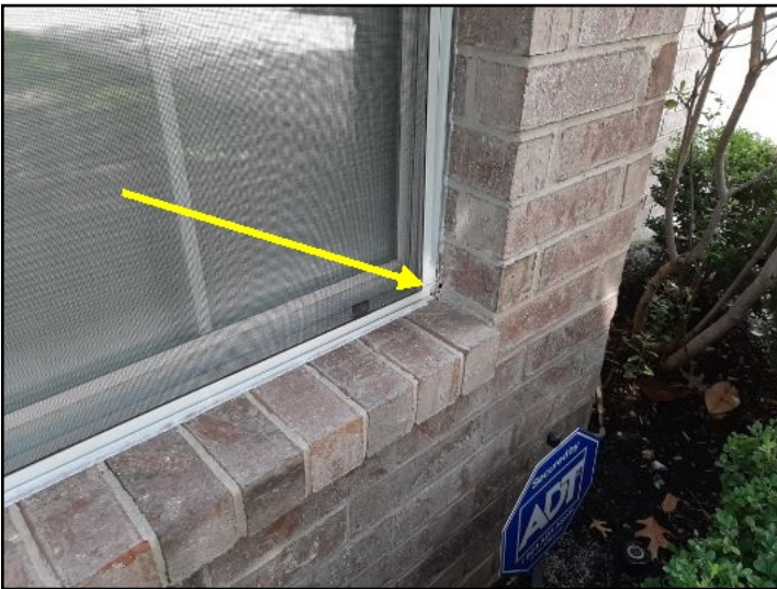
SEAL DETERIORATION
