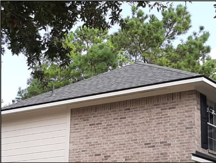
ROOF COVERING; LEFT
