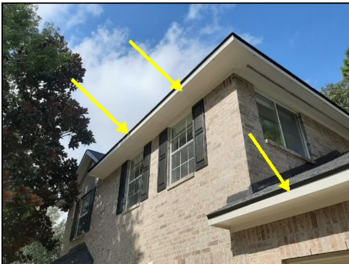
NO GUTTER SECTIONS
