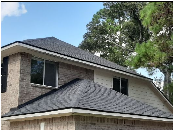
ROOF COVERING; RIGHT
