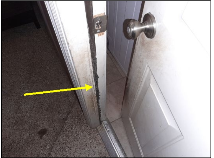
DAMAGED WEATHERSTRIPPING
