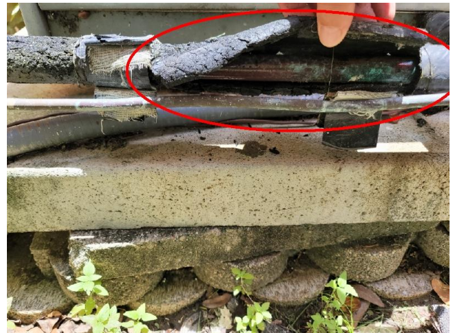
Damaged or missing insulation on the AC refrigerant lines at the condenser were observed. See the comments above
