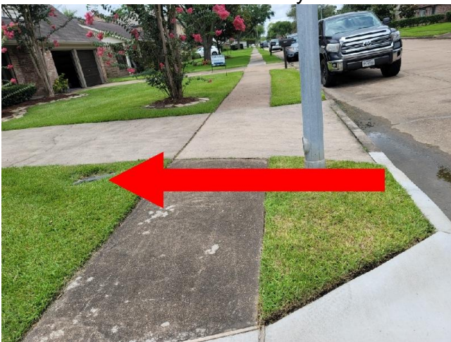
This Photograph confirms the location of the water meter within about 10" feet of the front curb.
