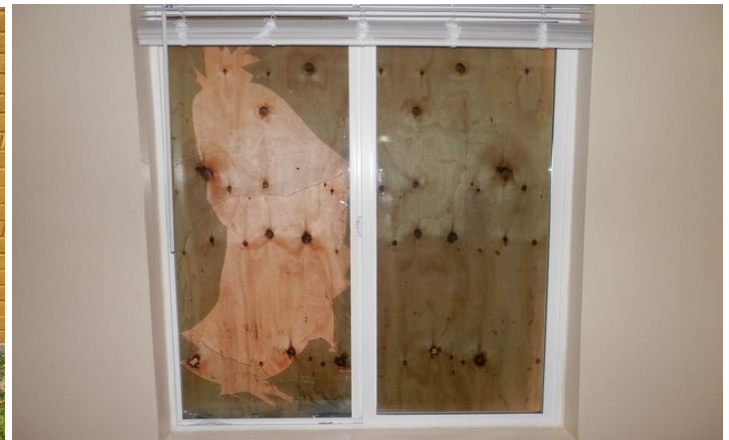
window covered at the outside, broken glass observed inside
