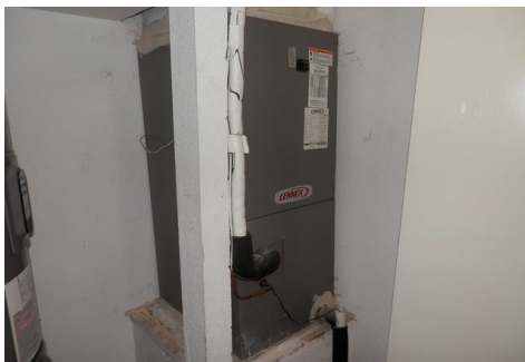
typical HVAC unit in the utility closet - checking heat output temperature in the test cycle (typical of all units)
