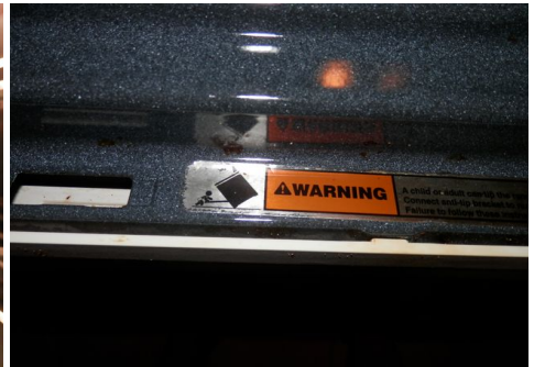
sample of cooktop and ovens in test mode - manufactures placard calling for an anti-tip device
