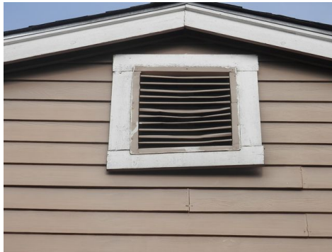
loose trim around the gable vent - general view of the back of the units
