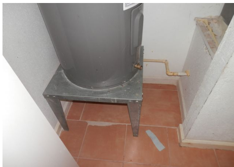
sample water heater (Unit A) without a drain pan - typical data plate for the 40 gal. water heater tanks
