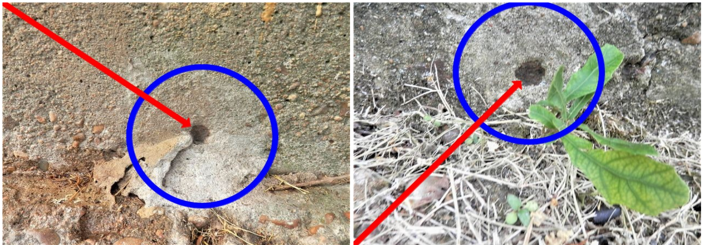
sample of exposed cable ends
