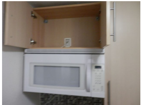
typical utility appliance installation - microwave with a recirculation type vent
