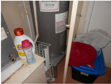
water heater in the utility area - data plate dated 2017 - sample of corroded supply line at top of water heater
