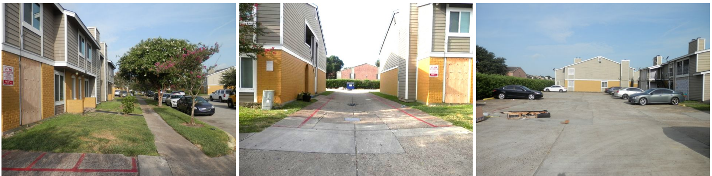
general view drain path at the front, left (driveway)
