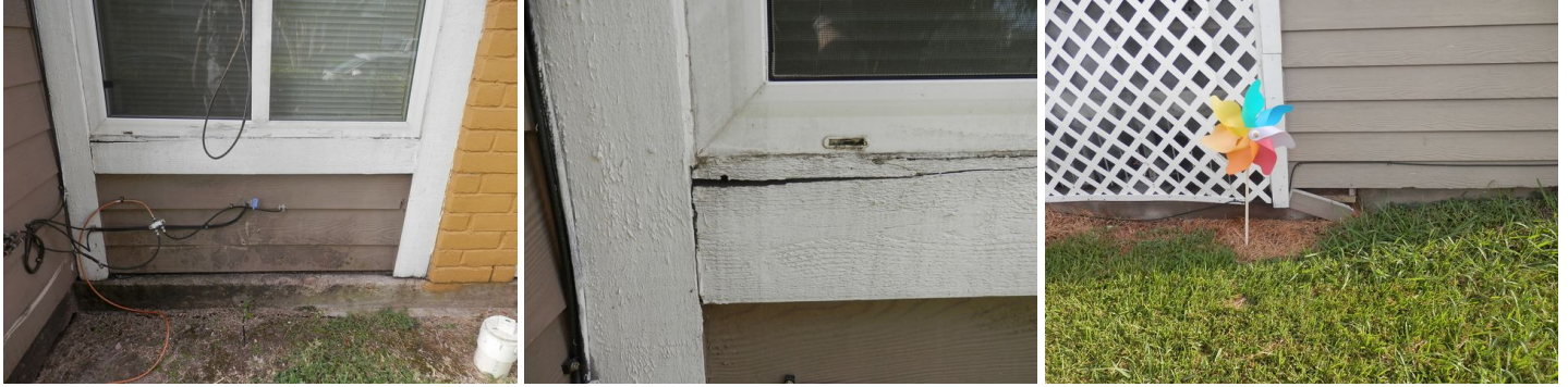
additional sample of voids in trim or loose trim
