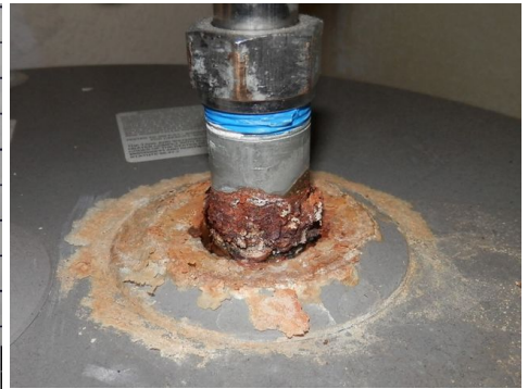
water heater in the utility area - data plate dated 2017 - sample of corroded supply line at top of water heater
