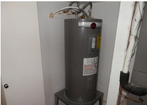
sample water heater (Unit A) without a drain pan - typical data plate for the 40 gal. water heater tanks
