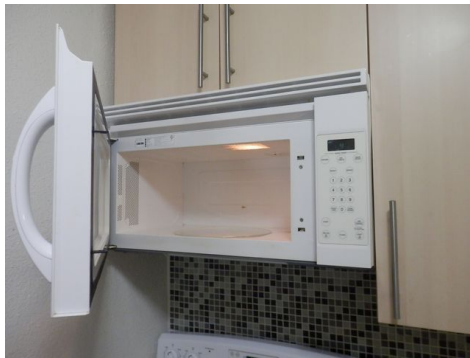
typical utility appliance installation - microwave with a recirculation type vent
