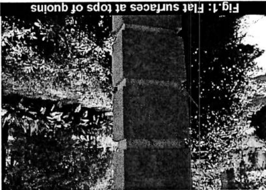
Fig. 1: Flat surfaces at tops of quoins
