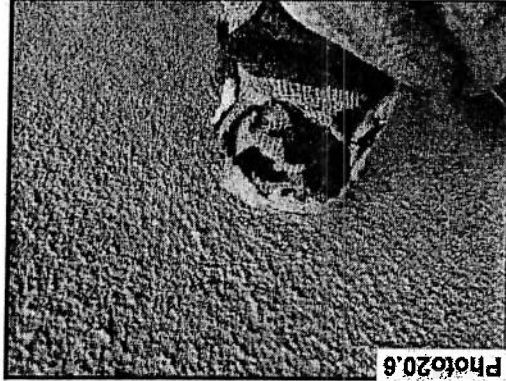
Casing bead trim to stucco panel transition, front elevation, sealant present but failing
