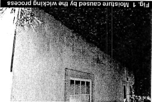
Fig. 1 Moisture caused by the wicking process
