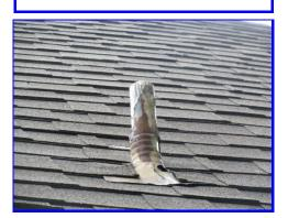
The lower front and upper front roof flashing is lifting - flashing repairs are needed
