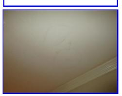
There is a large stress crack that radiates from the garage diagonally through the foyer and kitchen - foundation evaluation needed
