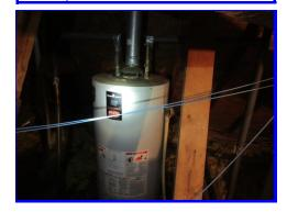
There is rust at the top of the water heater again heater replacement is needed
