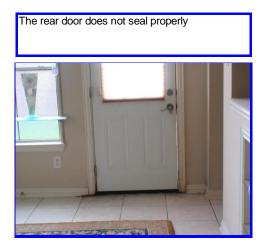
The rear door and door framing has significant water damage and will require full replacement
