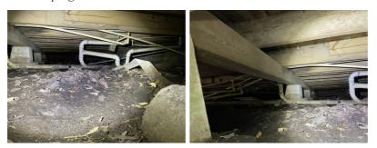
Drain Piping at Sinks: PVC Gas Supply Systems Present: Yes - Black Iron Areas of Rusting/Damage - Gas: No Water Pressure (PSI): 45 Specific Limitations: Note: Specific Limitations. The inspector is not required to:
