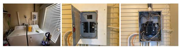
Electrical Service Entrance: Overhead Panel Location : Laundry Room Panel Brand: General Electric Main Conductor Wiring Type: Copper Panel Labeled?: Partially Panel Amps: 125 Amps
