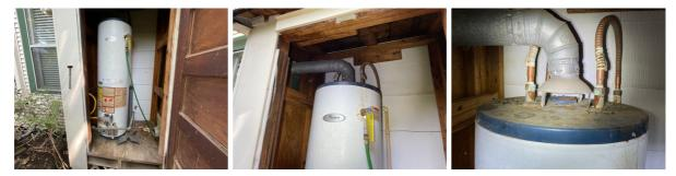
Energy Source: Gas WH Size: 40 WH Location: Exterior Closet TP Material: Galvanized Steel, Rubber hose WH Pan: No
