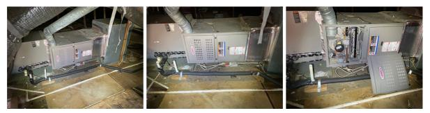
*Furnace Energy Source:* Gas *Furnace Type:* Forced Air - Gas Fired *Furnace Location:* Attic
