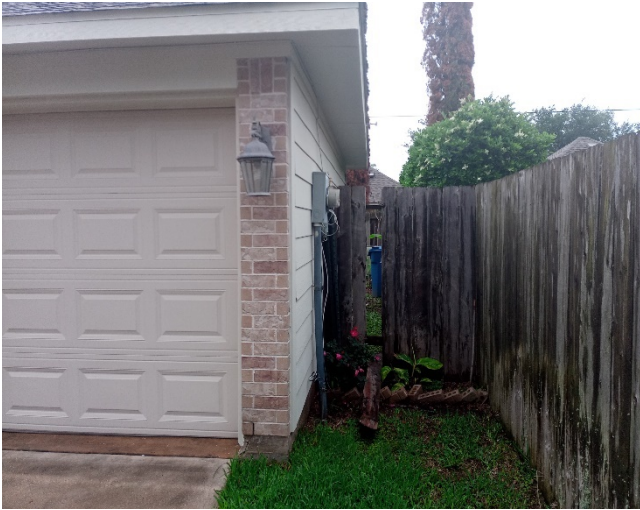
c. Backyard fence show signs of deterioration and have loose/leaning panels at various locations; recommend repair/replacement;
