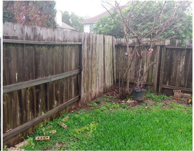
c. Backyard fence show signs of deterioration and have loose/leaning panels at various locations; recommend repair/replacement;
