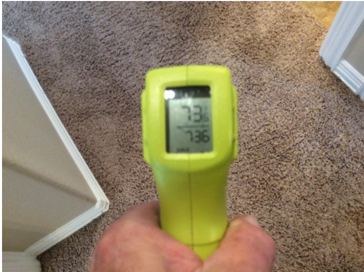
Upstairs heating return temperature 73°
