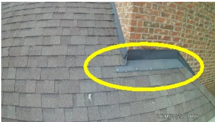
Exposed fasteners
