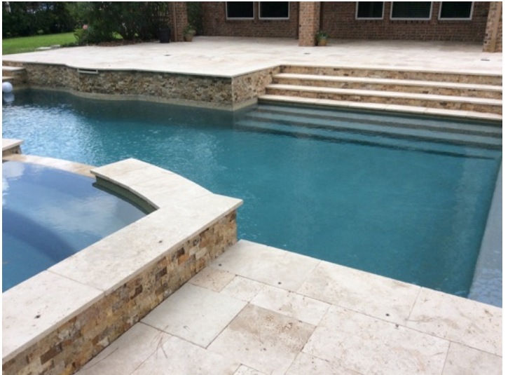
Pool, deck, and coping all appears in good condition
