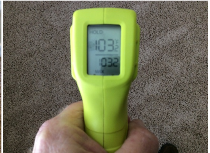
Upstairs heating supply temperature 103°
