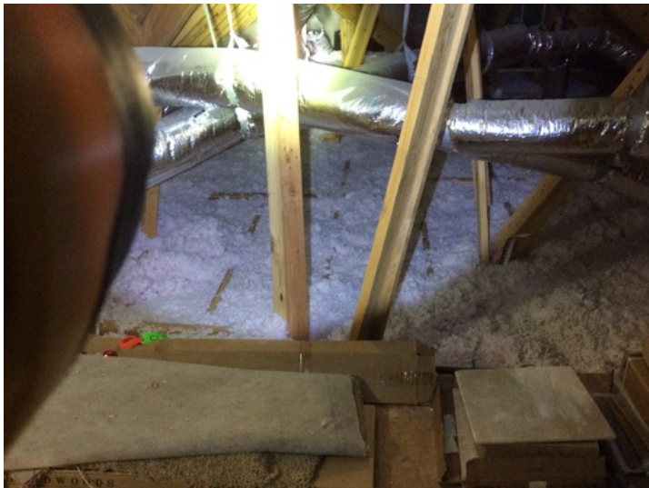
Blown in insulation
