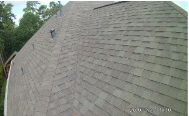
Various angles and views of the roofing system
