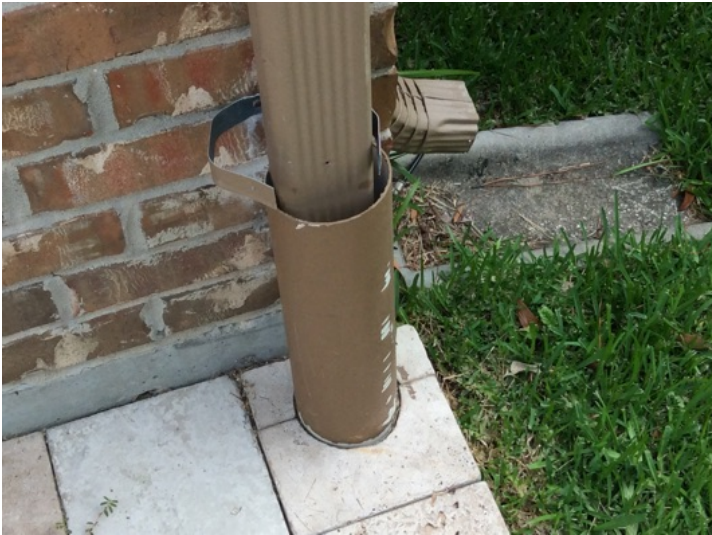
A strapping system for securing the downspouts to the underground drainage
