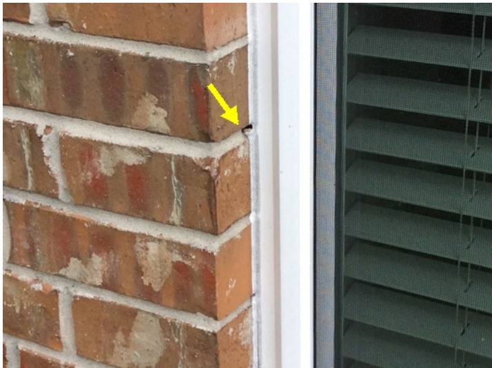
West wall observed wasps coming and going through this tiny hole near the window
