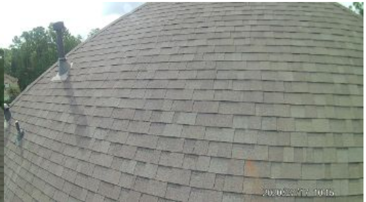
Various angles and views of the roofing system
