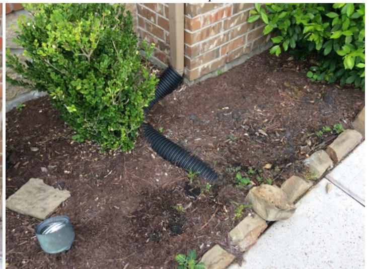
The gutter drainage system is tied into an underground drain system
