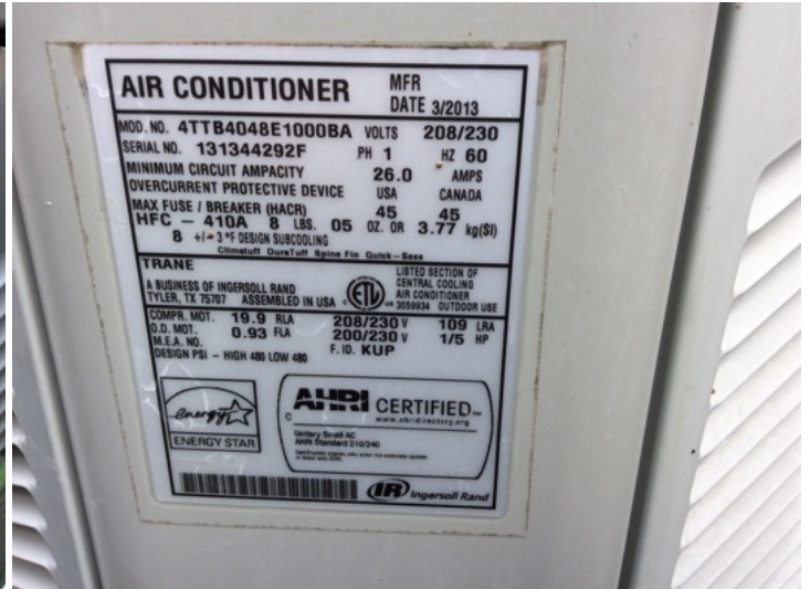
Trane air conditioner, 4 ton, manufactured March 2013
