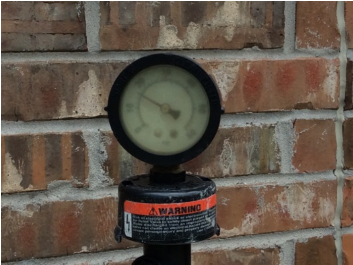
Operating pressure of the cartridge filter for the pool equipment is approximately 15 pounds PSI
