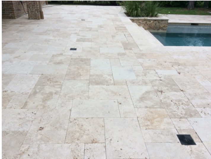
Pool deck with floor drainage appears to be in good condition
