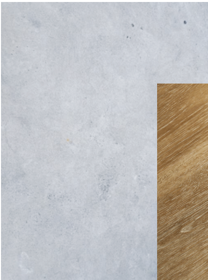
LIGHT CEMENT FLOORS (1ST FLOOR)
