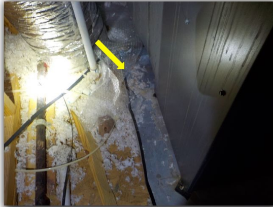
One evaporator suction line support strap is broken at the HVAC side attic.
