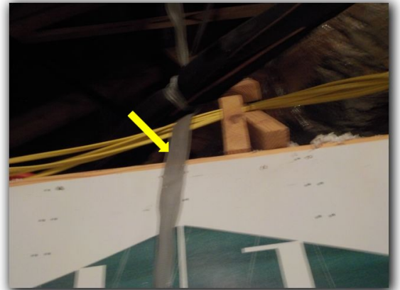
One evaporator suction line support strap is broken at the HVAC side attic.
