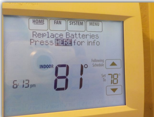
The upstairs thermostat has a low battery charge.
