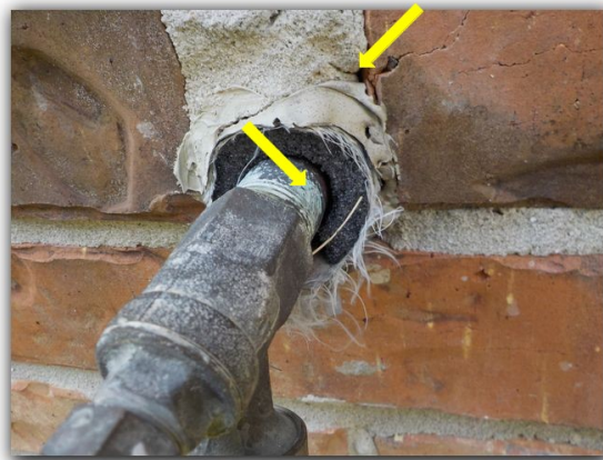
Wall piping penetrations should be sealed off.
