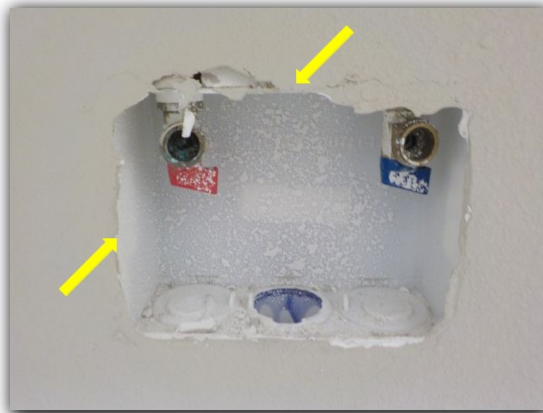
Wall piping penetrations should be sealed off.
