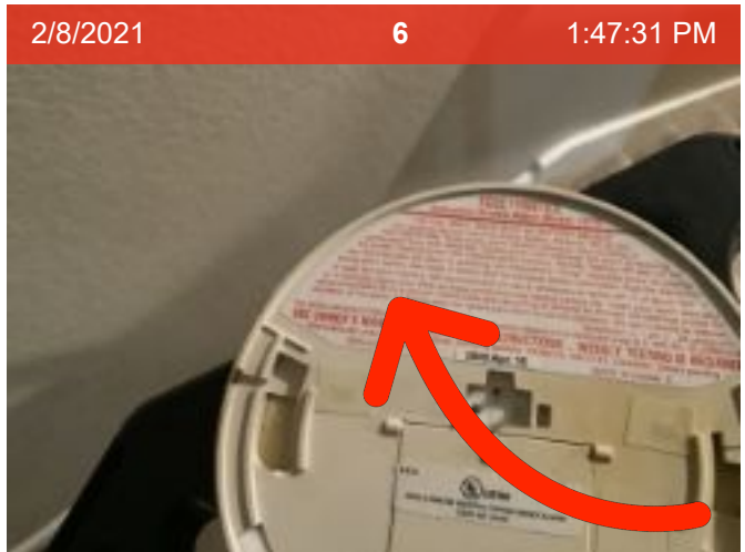
Wired Smoke Alarm (mfd 4/2005) | Smoke test: Passed | >10 yrs old | Close-up of printed manufacture
