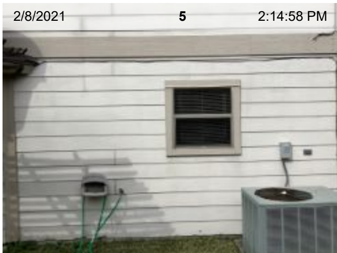
Walls/Siding/Trim | Left, Front, and Right Sides
