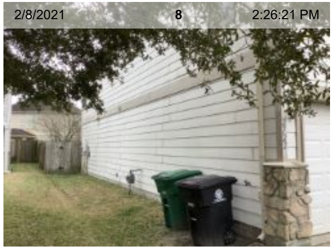
Walls/Siding/Trim | Left, Front, and Right Sides
