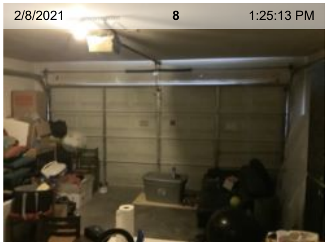
Garage Door Interior
