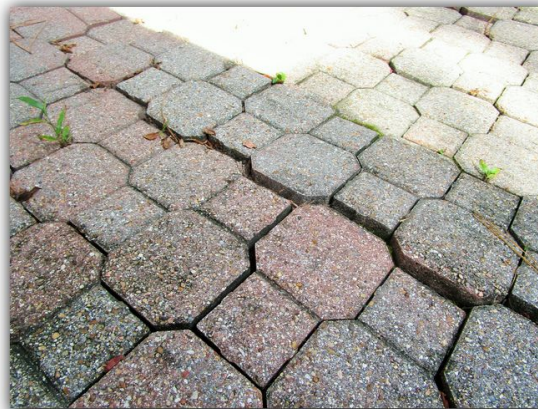
Walkway has heaving of slabs and cracks.
