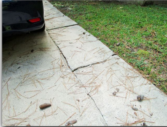
Uneven paver stones causing tripping hazard.
