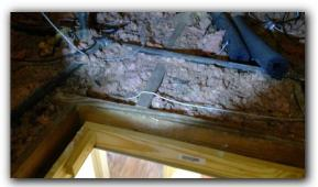
☑ Proper 30" working clearance and level platforms needed in front of equipment located in attic space at one or more locations.
