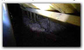
☑ Ridge board is not properly sized larger than the rafters attached per current standards and shows signs of movement.
