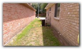
☑ Evidence observed of previous gutters present on house. It appears the gutters and downspouts have been removed, but downpout straps are still present in some locations.
