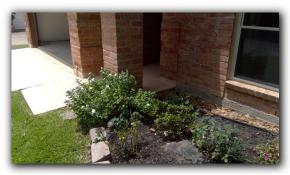
☑ Grade does not conform to current code requiring a 6" fall 10' from the structure
