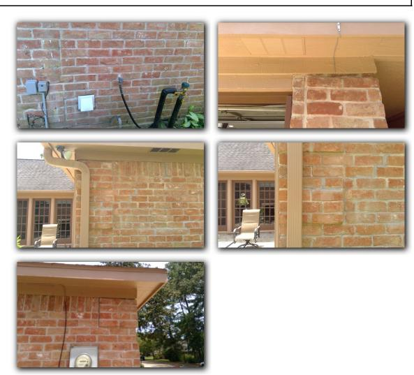
☑ Caulking / sealant is separated or missing in some areas
