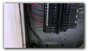
☑ Incorrect size of breakers / fuses: 20 amp is maximum size breaker that can be used on #12 wiring. 30 amp present
