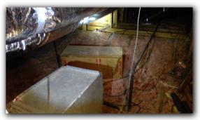
☑ Improper use of extension cords as permanent wiring observed in one or more locations. Permanent use of extension cords for permanent wiring is considered a safety hazard by current standards. See above microwave area.
