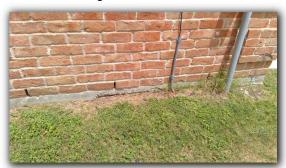
☑ Cracks observed in exterior brick walls showing some evidence that the foundation has moved / settled. (see exterior wall section for more pictures)
