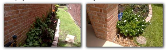
$\square$  Weep holes not properly spaced per current code standards at multiple locations. Current code requires a weephole within every 33".
