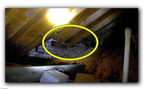
☑ Framing at attic access was cut and not properly supported at the hallway attic access..
