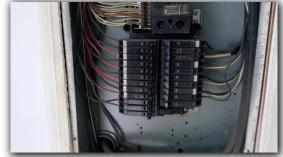
☑ Incorrect size of breakers / fuses: 15 amp is maximum size breaker that can be used on #14
