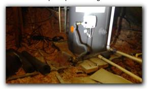
☑ 30" working clearance and platform needed in front of water heating equipment
