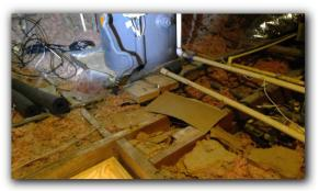
☑ Voids observed in insulation in attic space at one or more locations.
