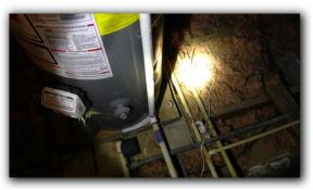
☑ Sediment trap not present in gas line at water heating equipment
