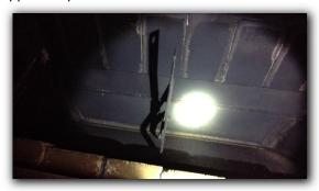
☑ Gas valve does not require the use of a separate key. This can present a potential safety hazard if valve is turned without the use of the key and gas is inadvertantly turned on.
