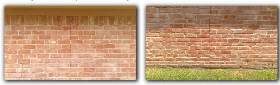
${\ensuremath{\overline{\square}}}$  Evidence of previous exterior siding repairs observed
