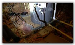
Attic does not conform to current code requiring a continuous / solid and unobstructed 24" wide catwalk
