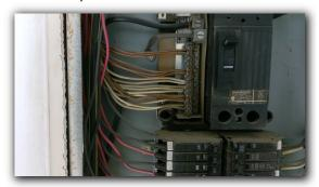
☑ Lack of anti-oxidants on aluminum conductor terminals in panel box at one or more locations.
