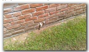
☑ Water heater T & P valve piping is plumbed with wrong material. Piping present is not rated for hot water use.
