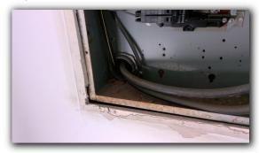
White "neutral" type wiring used as "hot" needs to be properly identified as "hot" in panel box at one or more locations. White wiring should be wrapped with black tape or marked with a black (or other appropriate color that is not white, grey or green) marker.
