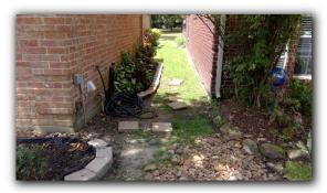
☑ Drainage on the left side of the house does not appear to be properly draining water away from the foundation
