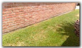
☑ Soil level too high around the front porch post (s) areas at one or more locations. Grade does not conform to current code requiring a 4" slab exposure between the finished grade and exterior brick
