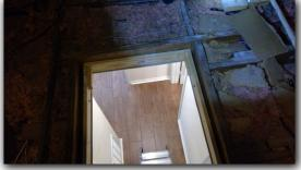
☑ Framing at the attic access does not conform to current standards requiring double framing for the access door.
