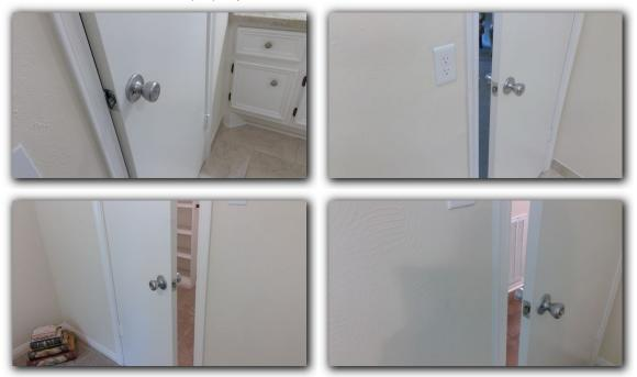
☑ Ball latches appear to be damaged / missing at one or more door locations which keeps the door from latching properly. See study closet area. Doors do not appear to be supplied with appropriate ball latches.
