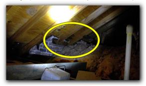
☑ House was not constructed per current standards requiring the purlin brace to be the same size or larger than the rafter being supported. 2 x 4 purlins supporting 2 x 6 rafters observed.
