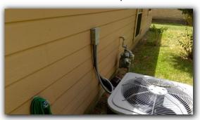
lackimsquare Conduit is not properly connected / installed at exterior wall
