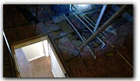
☑ Cut framing around the fireplace chimney does not appear to be properly supported..
