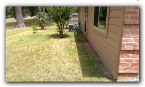
☑ Drainage on the right side of the house does not appear to be properly draining water away from the foundation
