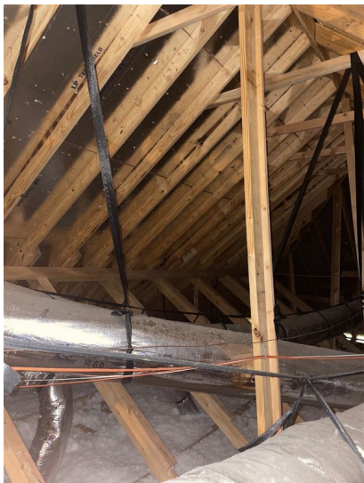
Approximate Average Depth of Insulation: 12 Inches
