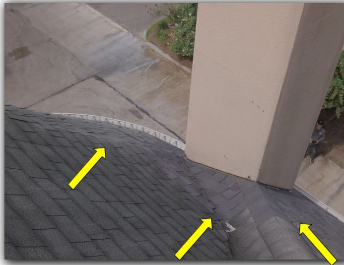
Observed spot repairs to roof surface.(Around the chimney)
