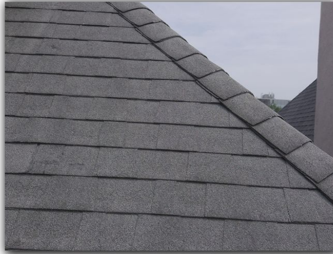
Observed spot repairs to roof surface.(Around the chimney)
