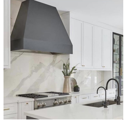
Kitchen Vent Hood
