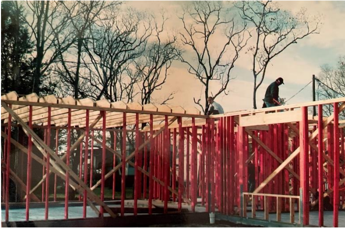
4118 Grand Boulevard Construction photos supplied by homeowner.
