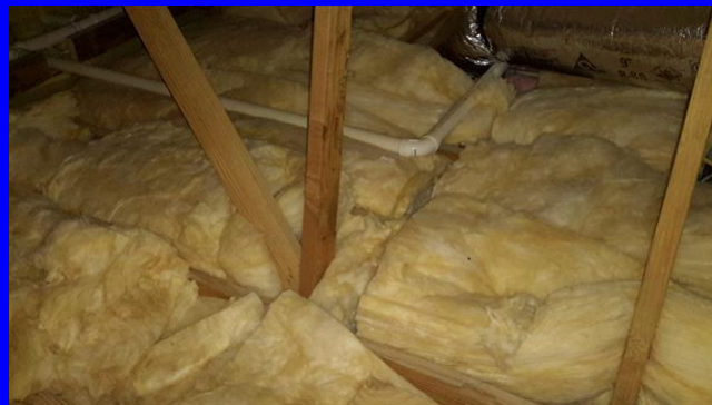
10 to 12 inches of batt insulation in the attic
