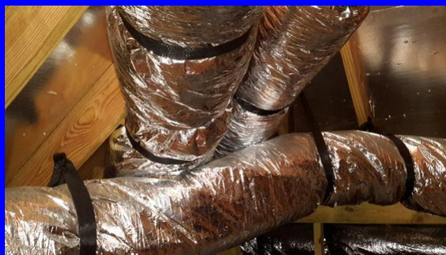
insulated ductwork
