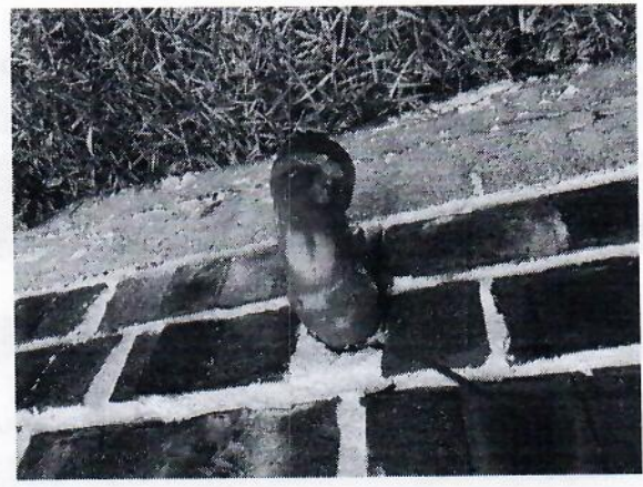
Utility room floor drain not sealed at wall
