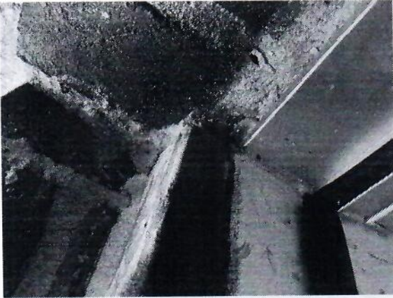
Caulk missing at rear patio door jamb at base
