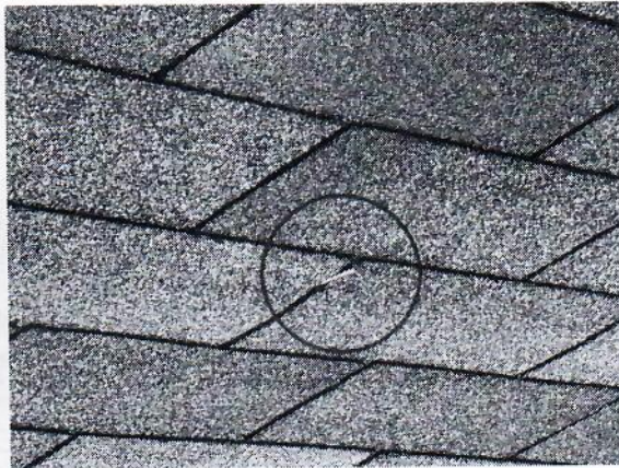
Loose nails at roof covering
