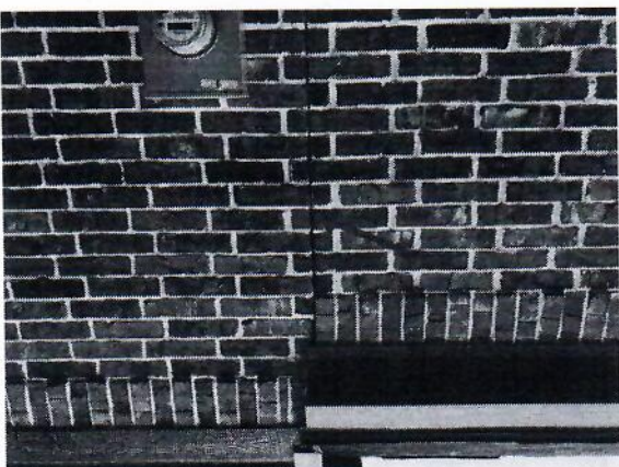
Mortar crack above garage door
