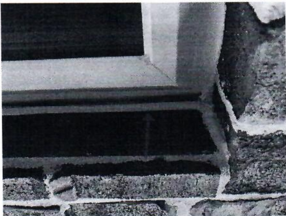
Expansion joint caulking missing exterior walls
