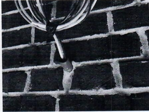
Hose bibs not sealed at exterior walls
