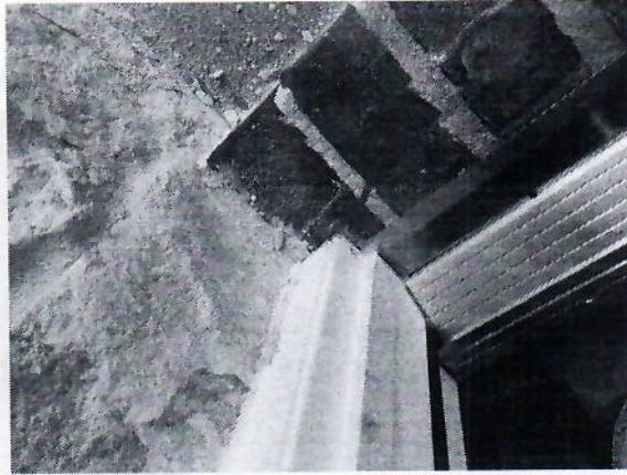
Paint missing at rear patio door jamb
