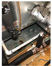
2- Installed missing pipe insulation causing condensation dripping, no more moisture noted
