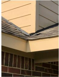
3- Removed debris from under shingle, now lays flat
