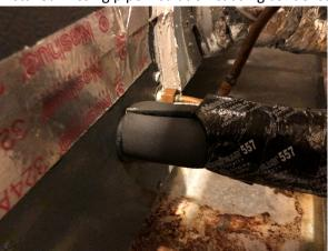
3- Replaced refrigerant pipe insulation
