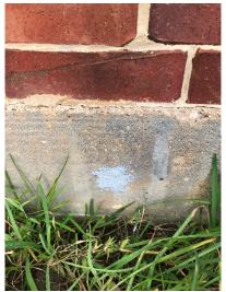
2- Sealed cracks on edges of foundation
