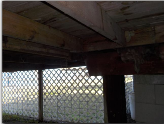
Wood rot and/or deterioration was observed at the bottom of various piers supporting the foundation for both porches.
