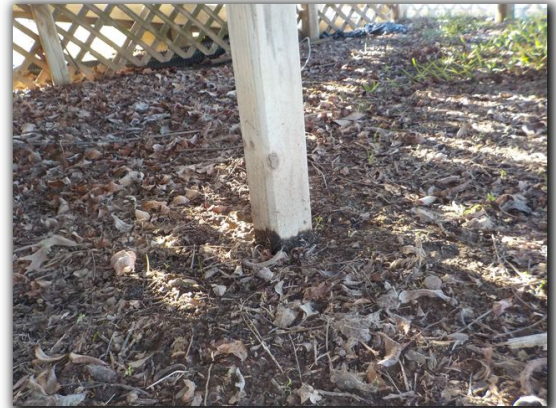
Wood rot and/or deterioration was observed at the bottom of various piers supporting the foundation for both porches.
