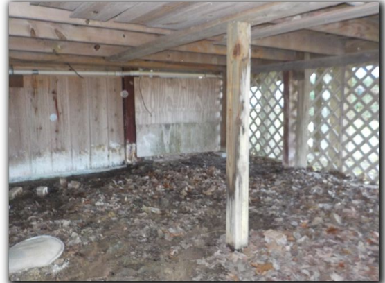
Wood rot and/or deterioration was observed at the bottom of various piers supporting the foundation for both porches.
