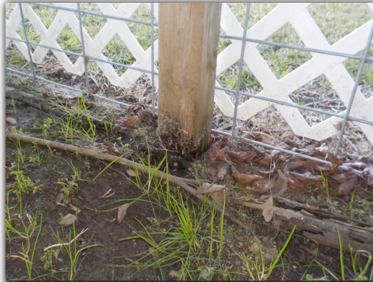
Wood rot and/or deterioration was observed at the bottom of various piers supporting the foundation for both porches.
